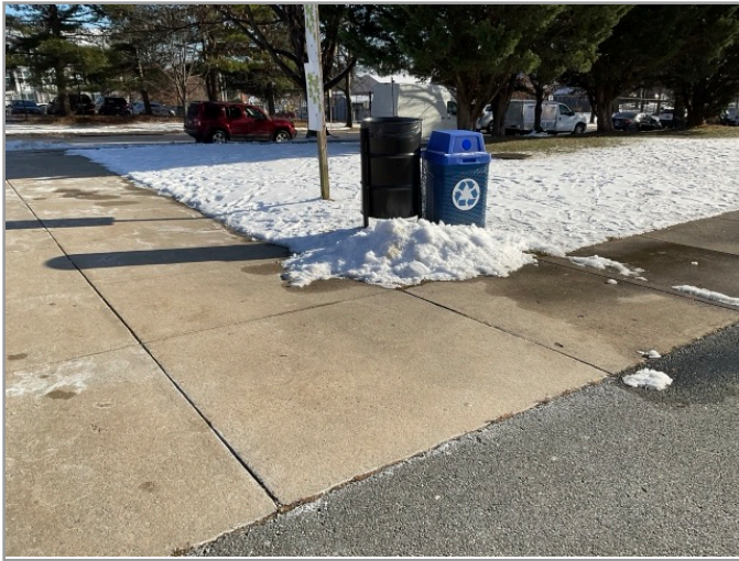
ACCESSIBLE ROUTE TO PLAYGROUND
