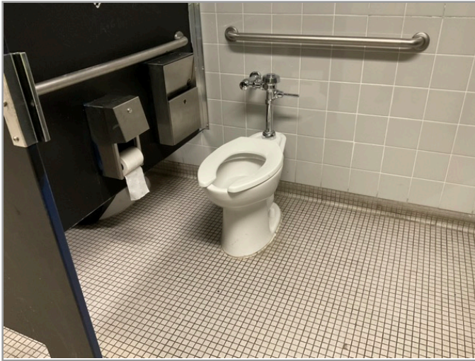
TOILET STALL OVERVIEW
